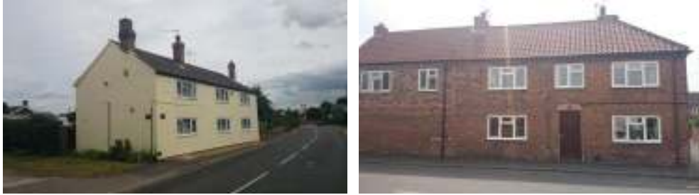
Figure 4.9: The row of former cottages on Top Street (left) has been irrevocably altered, the original (18 th /early-19 th century) doorways and window openings no longer being visible and the wide openings and render resembling a 1950s property. The building on the corner of High Street and West Street (right) has seen all of its window openings enlarged and a doorway partially infilled, again giving a 1950s appearance. Of particular note is the new window opening overlapping the old doorway on the front, giving an untidy appearance at odds with the character of the historic building.
