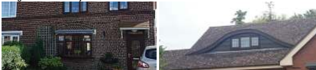
Figure 3.22: Brick detailing at Top Street (left) and eye-brow dormer on Slaynes Lane (right).
