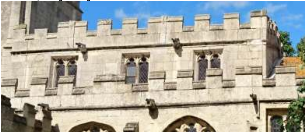
Figure 3.6: Clerestory openings, south side.
