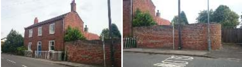
Figure 4.1: Northfield Farmhouse, railings and wall.
