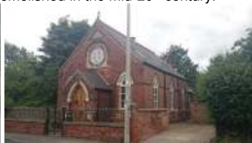
Figure 2.7: Former Wesleyan Methodist Chapel, built 1897.
