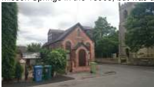
Figure 2.6: Former Primitive Methodist Chapel, built 1873.
