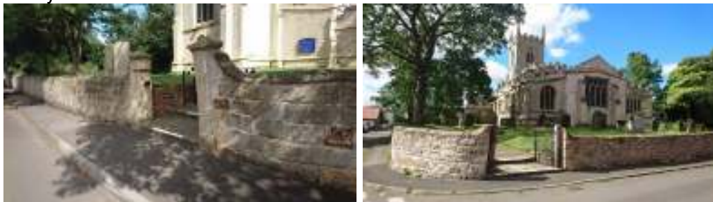
Figure 3.28: Stone boundary wall around the churchyard.
