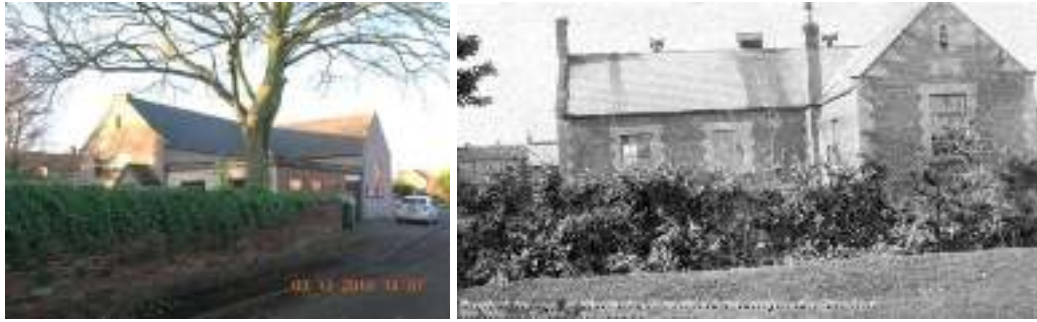
Figure 3.18: Former village school, now village hall, including from 1920 (source: www.picturethepast.org.uk , accessed 2017).
