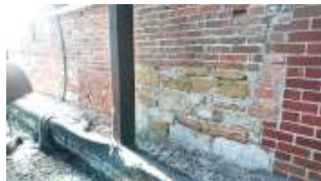
Figure 3.25: Section of earlier stonework within 18 th century barn at Gibdyke Farm.
