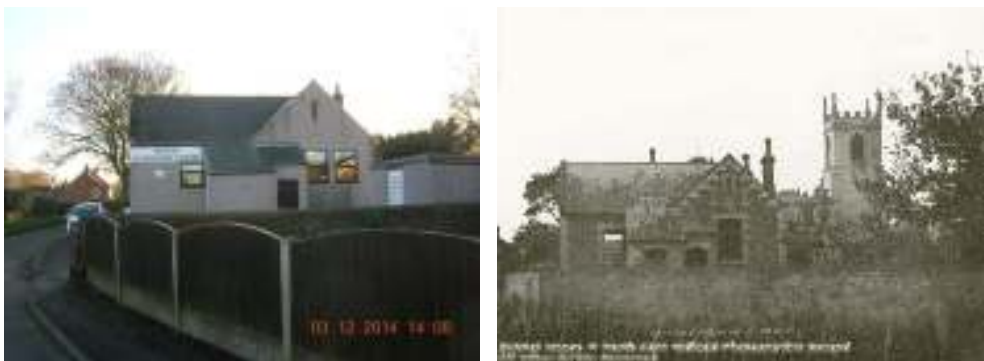
Figure 4.5: The addition of a pebbledash render onto the former school, now Misson Community Centre, covered over the two-tone red and yellow brick detail of the building, a key part of its Victorian character. This change, together with the loss of chimney stacks, installation of unsympathetic windows and doors and the addition of a flat roof extension have all exacerbated the harm.
