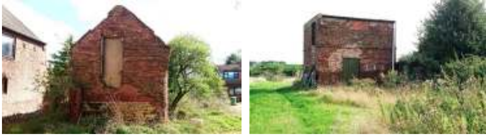
Figure 4.3: Former agricultural buildings on Top Street (left) and Gibdyke (right), both in a state of disrepair. The building on Top Street is unusual with its stone plinth facing the road, although its overall condition detracts from its significance. The structure at Gibdyke has also seen its original roof lost and other unsympathetic changes.
